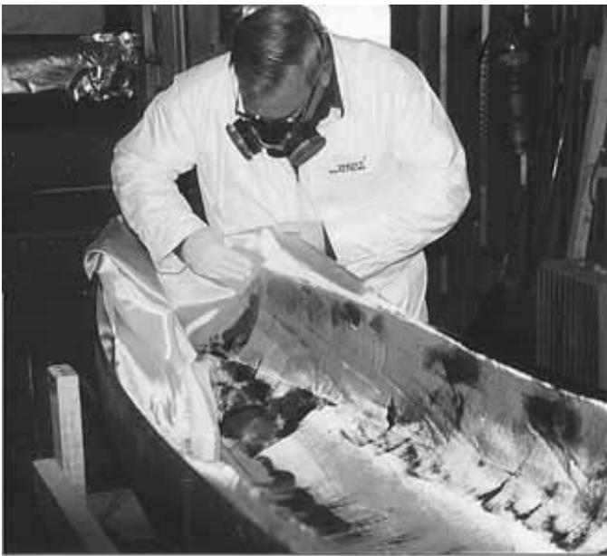
Installing Layer One Of Glass
